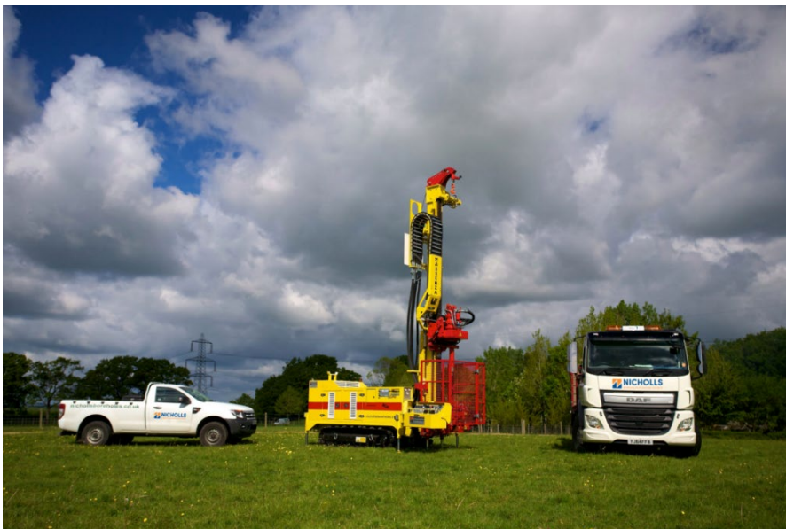
Image: A standard bore rig with drill and support vehicle.
