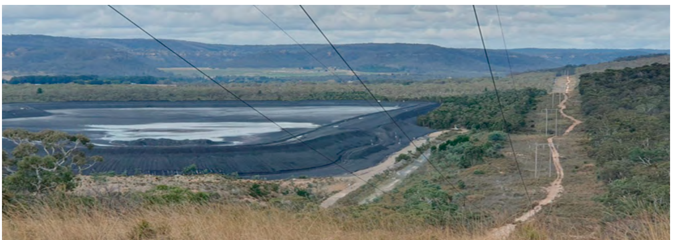
Image: Photo of current 45 m easement for 132 kV transmission line. Under the preferred route option, Transgrid is proposing to increase the width of the easement by approximately 15 m to the north (left hand side) to accommodate the new 330 kV transmission line. The 330 kV line would replace the 132 kV line shown above.
